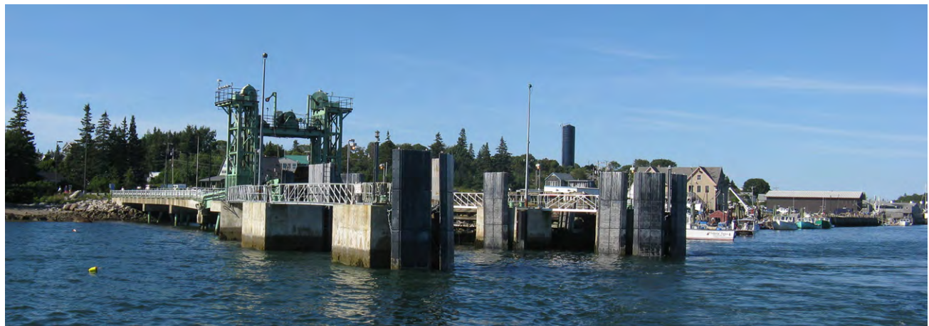
Vinalhaven ferry terminal.
