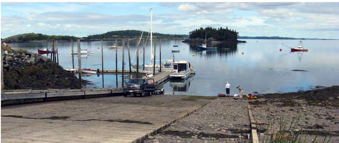
The concrete boat ramp: the only ramp in town capable of handling larger fishing vessels, shown here at low water.
